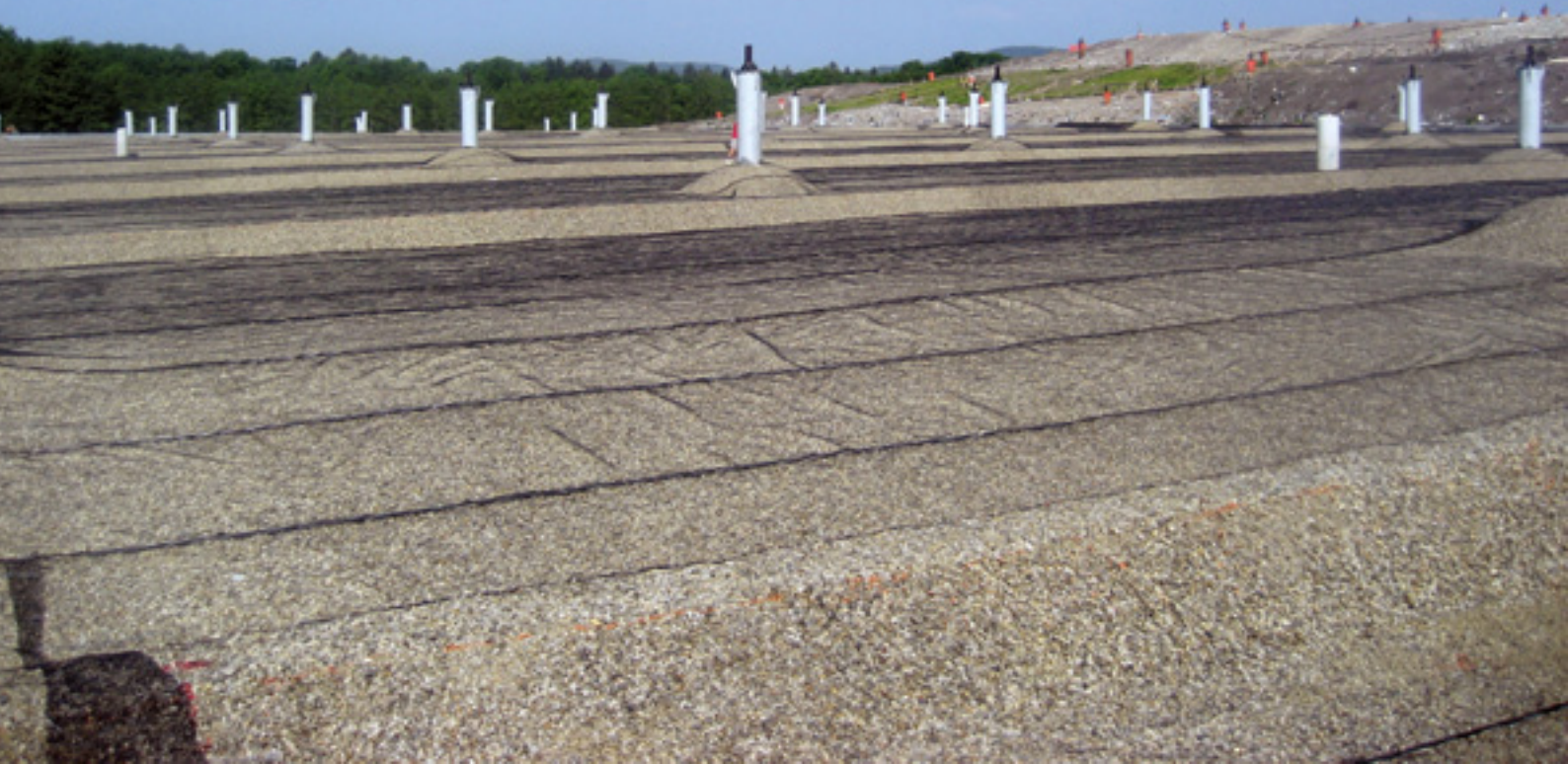
Upgrade of the Ljubljana Regional Waste Management Centre (RCERO), Ljubljana, Slovenia Area: 49 289 m 2 , maximum capacity of waste: 884 681 m 3 , location: Ljubljana Barje. Refer to page 64.
